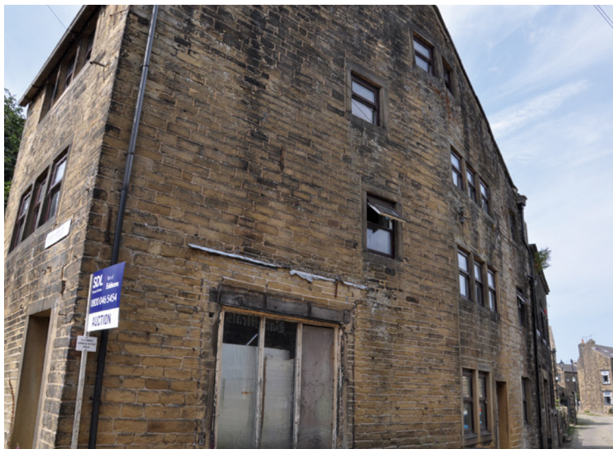
The newly-acquired historic buildings on West Lane in Haworth.
